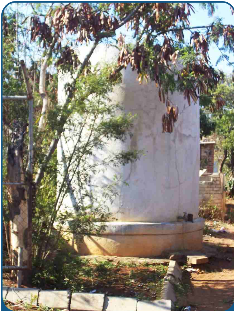
Rain Water Harvesting Concrete Containers
